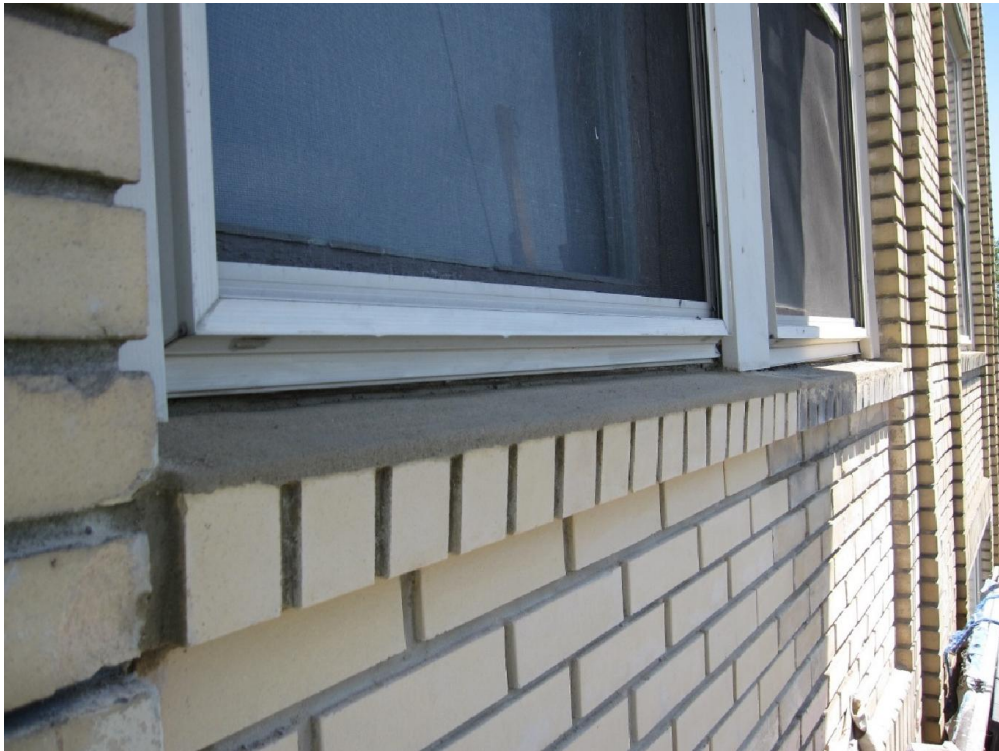
figure no.17: Completed air conditioner opening restoration.
