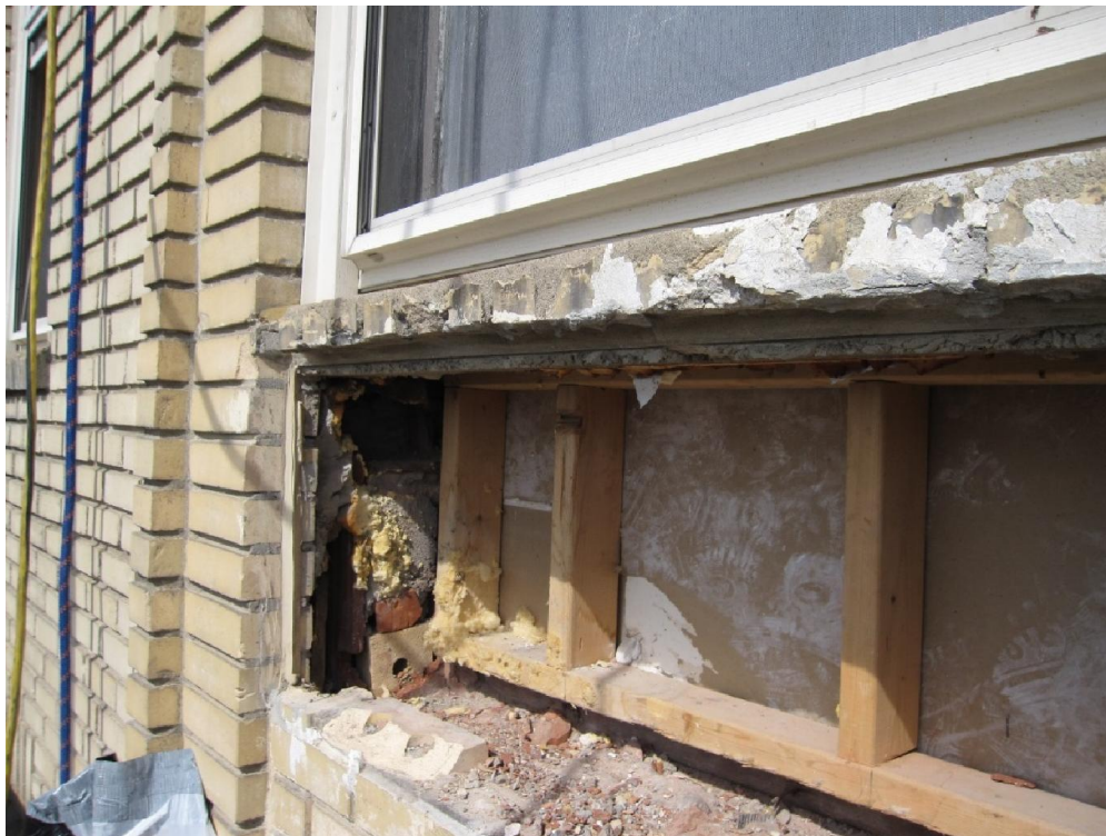
figure no.7: This was an A/C opening that was abandoned in place in Unit F5. The picture is after removal of the grate and a foam board that was held in place with expandable foam.
