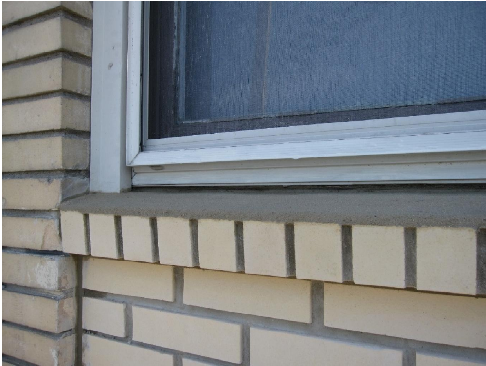
figure no.16: Sill cap course with the mortar top coat
